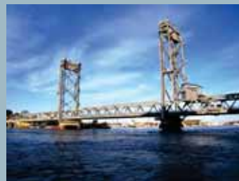
2013 Memorial Bridge. Photo: NHDOT
