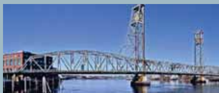
Historic: Memorial Bridge, constructed 1923. Courtesy of John White and Steven Smith, Portsmouth Preservation
